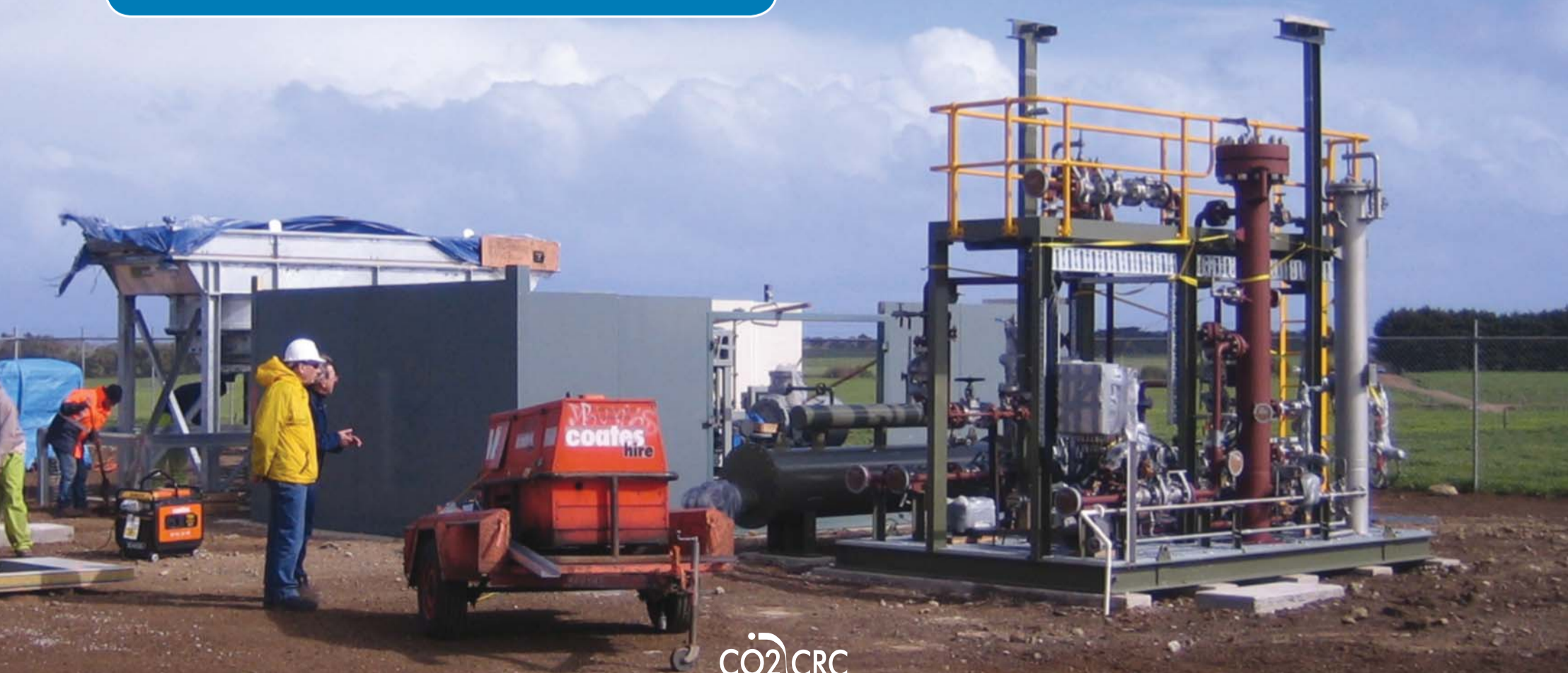
Above: surface plant and production well, process skid, compressor.
